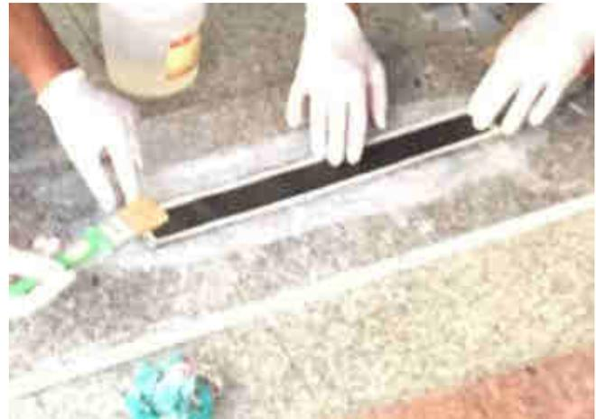
Fig. 4.6: Applying of resin over each ply
