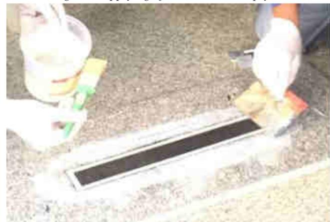
Fig. 4.7: Removing of air bubbles
