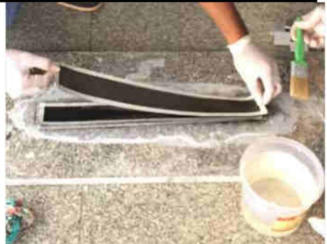
Fig. 4.5: Placing of one ply of CFRP over another
