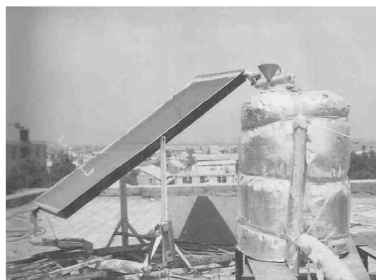
Fig. 2: The Solar Water Heating System Used in the Study
