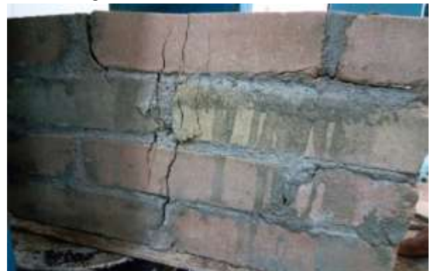
Fig.12: Crack Pattern (Parallel to Bed Joint)
